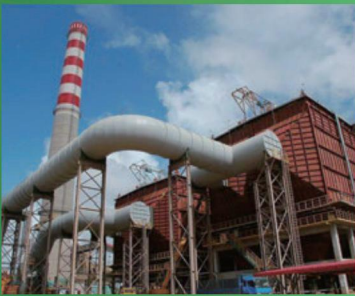
Electrostatic precipitator
