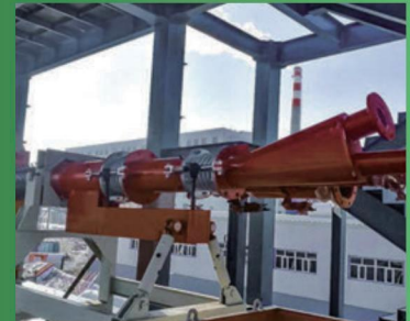
Four-channel pulverized coal burner
