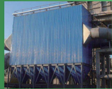
Plate electrostatic precipitator
