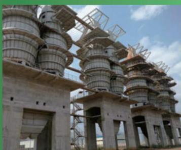
Double-chamber lime kiln
